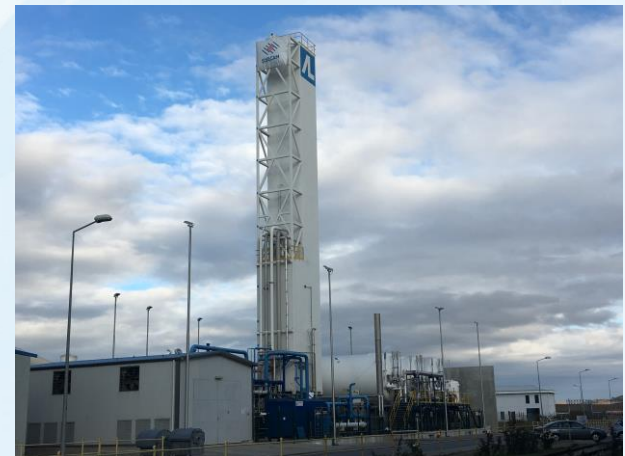
Air Liquide O 2 & N 2 plant
