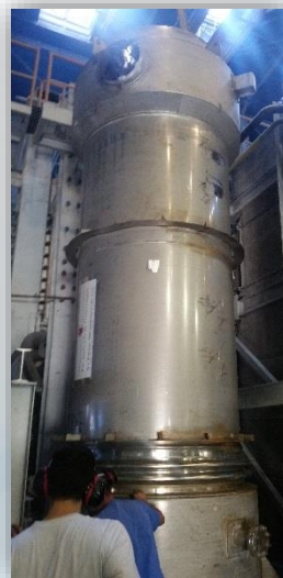
Recuperator installation
