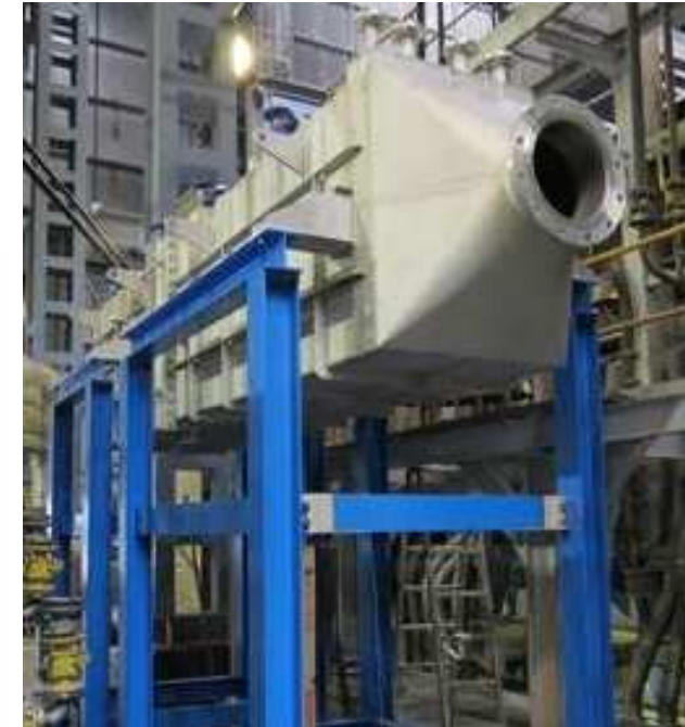
Secondary heat exchanger during installation
